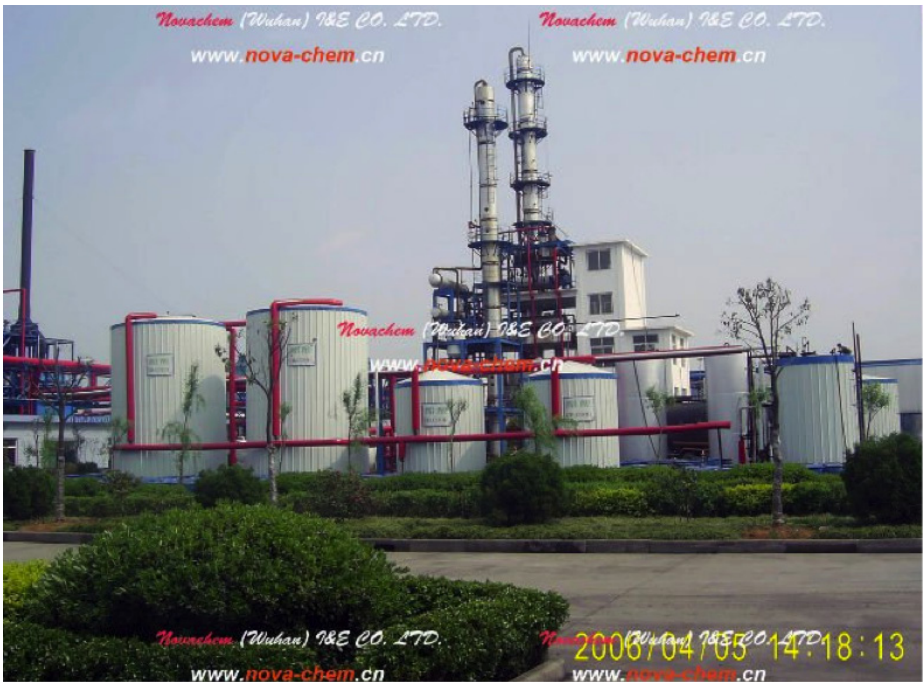
The Novachem (Wuhan) Import & Export Company Ltd. Vitamin C Manufacturing Facility in China
